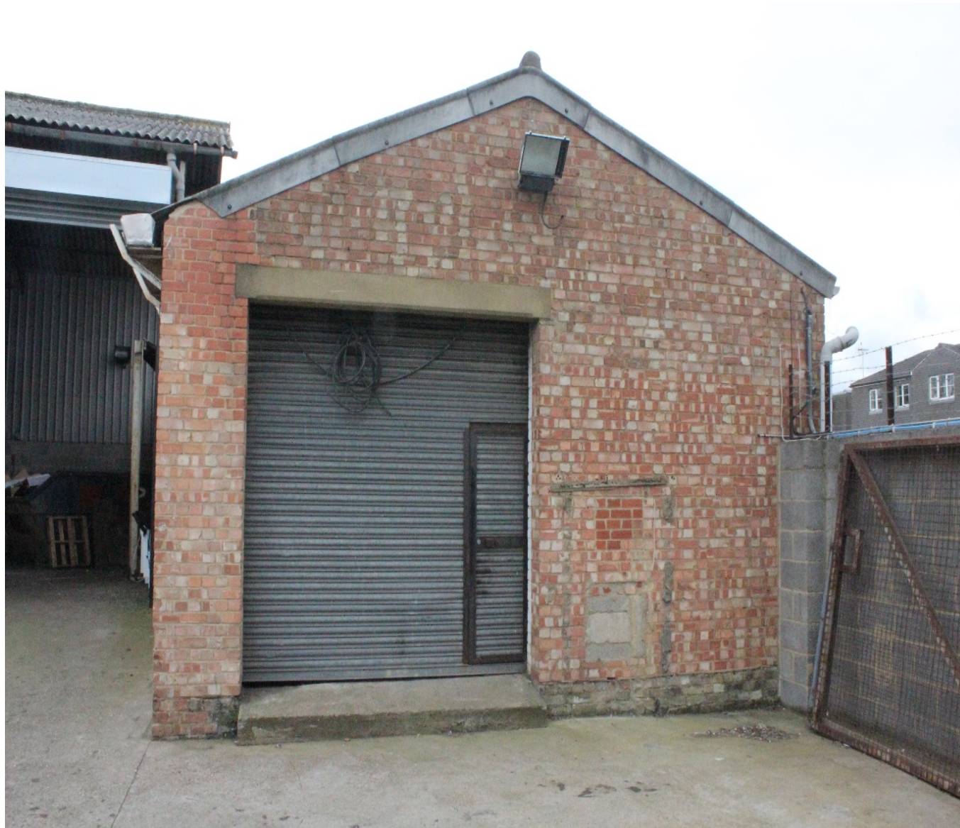
Plate 11: Northern end of the south western outbuilding (facing SW)
