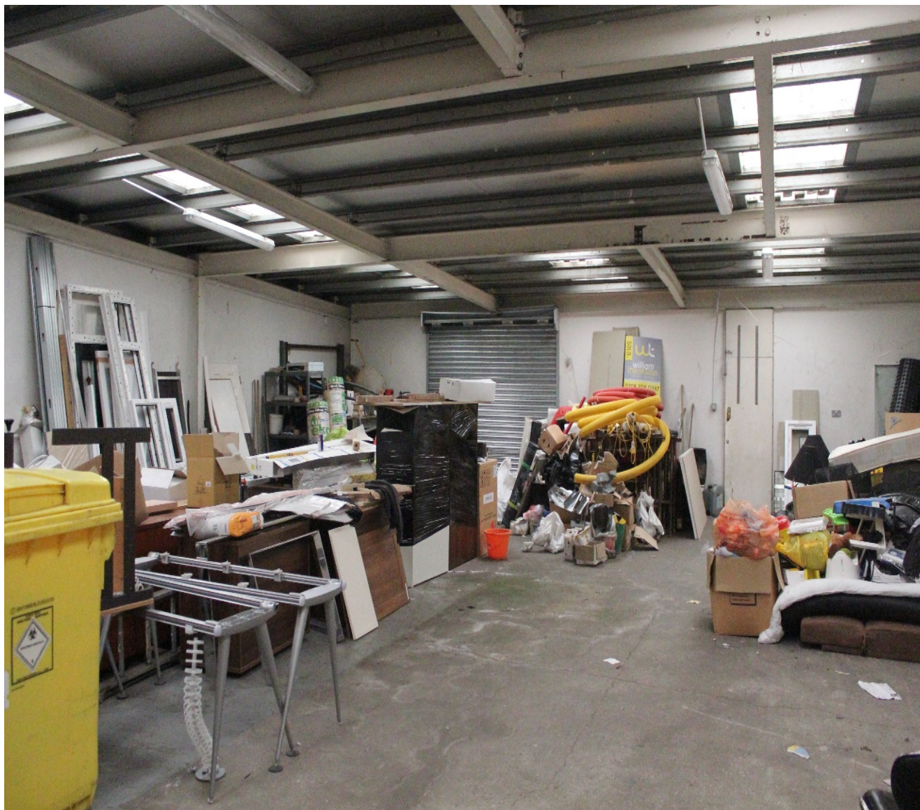
Plate 7: Looking across the rear single storey extension (facing SSE)
