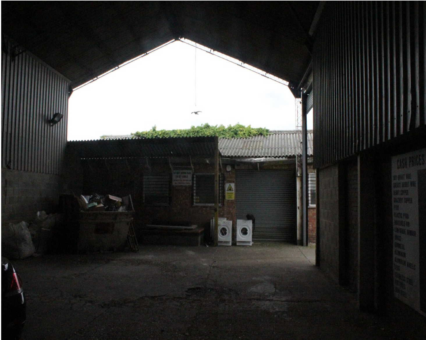
Plate 8: View towards the yard access and the south western outbuilding (facing WNW)
